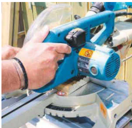
STEP 2. Cut all the deck boards to length using the miter saw, or by hand if you don't have one
